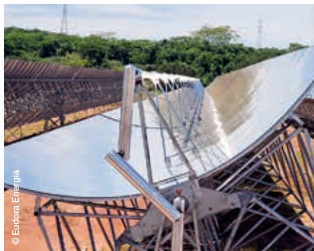
Five arrays of parabolic troughs heat up a thermal fluid to 350°C (662°F).
