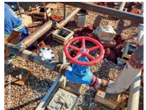
KVN piston globe valves are a vital part of the green energy project.
